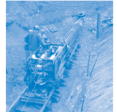
CUC employees put in a horizontal bore near College Road.
