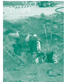
GHU employees water distribution maintenance.
