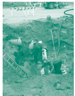
GHU employees water distribution maintenance.
